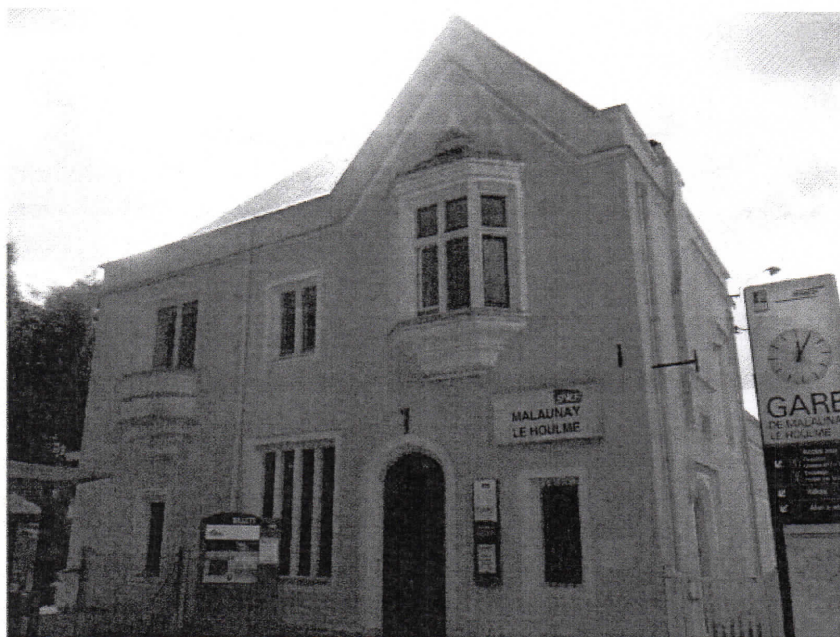
2. Malaunay railway station, designed by William Tite, 1843. Photograph by the author.
