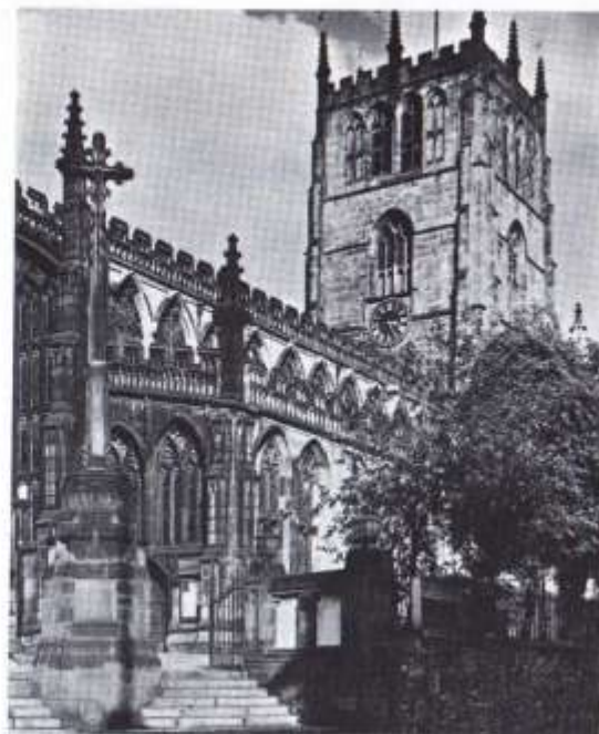
Parish Church of St. Mary the Virgin, Nottingham. In existence since Saxon times, it is now mainly a 15th Century structure. In this church Hiram's parents were married on 1st August 1795.
