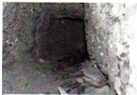
The Tunnel from the cellar
