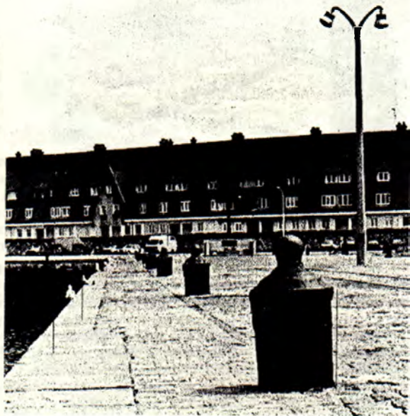
The Courgain in 1996. The barricade posts are made of upturned cannon barrels.
