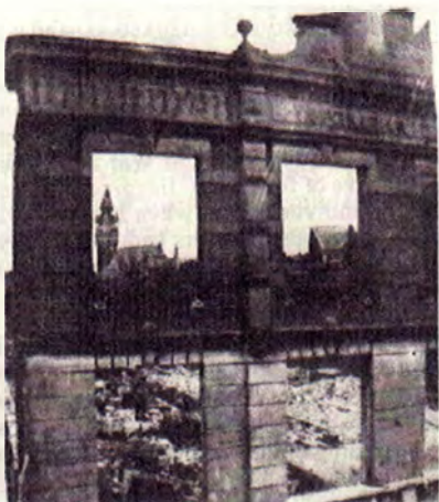
Factory of Vampouille & Duquesnoy, rue des Quatre Coins, totally destroyed by the first British bombs on 15.09.40. Photo R Chaussois - from Les Calaisens et la dentelle 1906/1950 . M Caron
