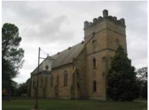
Figure 1: St James Anglican Church, Morpeth (Photo RJL)
